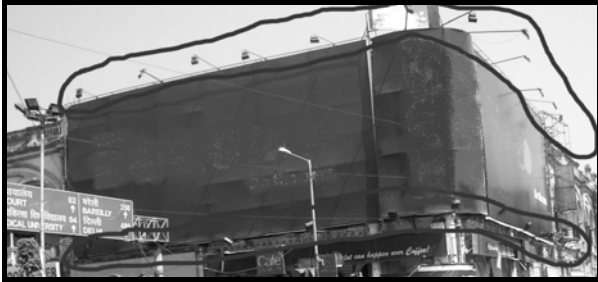
Figure 3. A big sized hoarding with a large number of illumination lamps.
